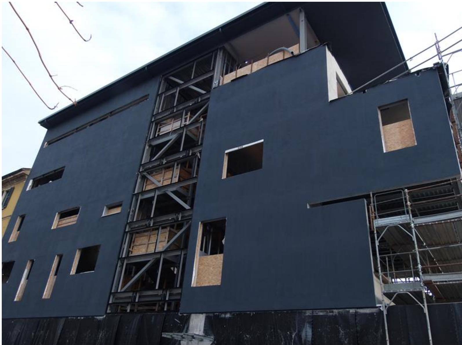
COMPLETAMENTO FACCIATA A SECCO SU STRADA CON FINITURA CON INTONACO COLORATO IN PASTA CONNI DI KNAUF
