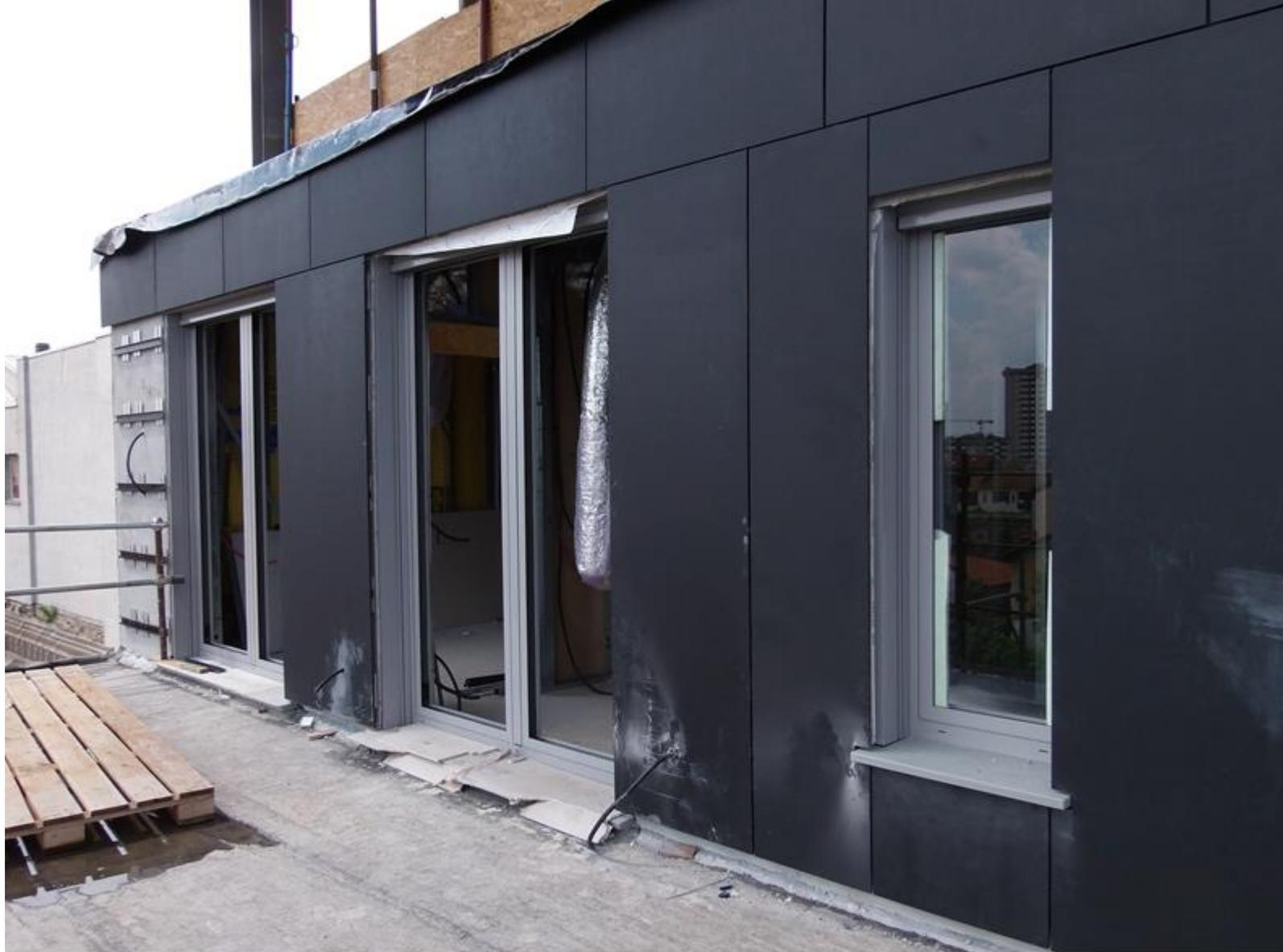
**MONTAGGIO DI PANNELLI IN GRC. USCITA CORRUGATI ELETTRICI CON TAPPI IN GOMMA A TENUTA ALL'ARIA**
