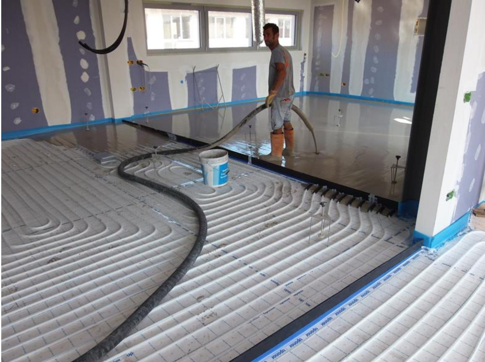
POSA DI PAVIMENTO RADIANTE UPONOR KLETT E MASSETTO FLUIDO AD ALTA EFFICIENTA DI 4 CENTIMETRI DI SPESSORE KNAUF FE 80
