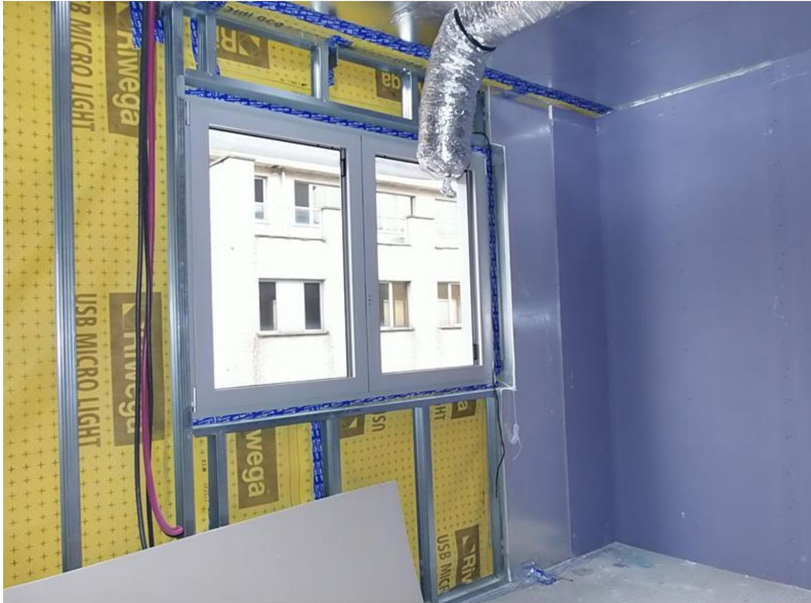
PARTICOLARE CHE EVIDENZIA LA LASTRA DI FINITURA INTERNA CON BARRIERA AL VAPORE E LASTRA DIAMANT DI KNAUF
