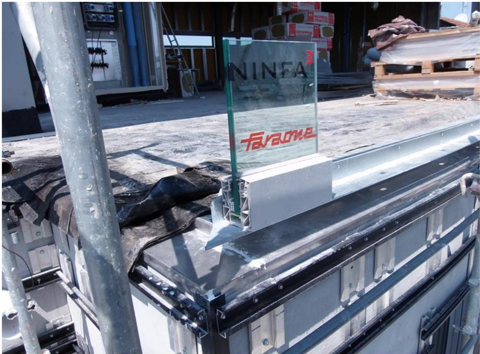
PROFILI IN ACCIAIO ZINCATO SU MISURA A "Z" PER IL SOSTEGNO ED IL FISSAGGIO DEI PROFILI IN ALLUMINIO NINFA 3 FARAONE PORTA PARAPETTI IN VETRO PER I TERRAZZI A TUTTI I PIANI
