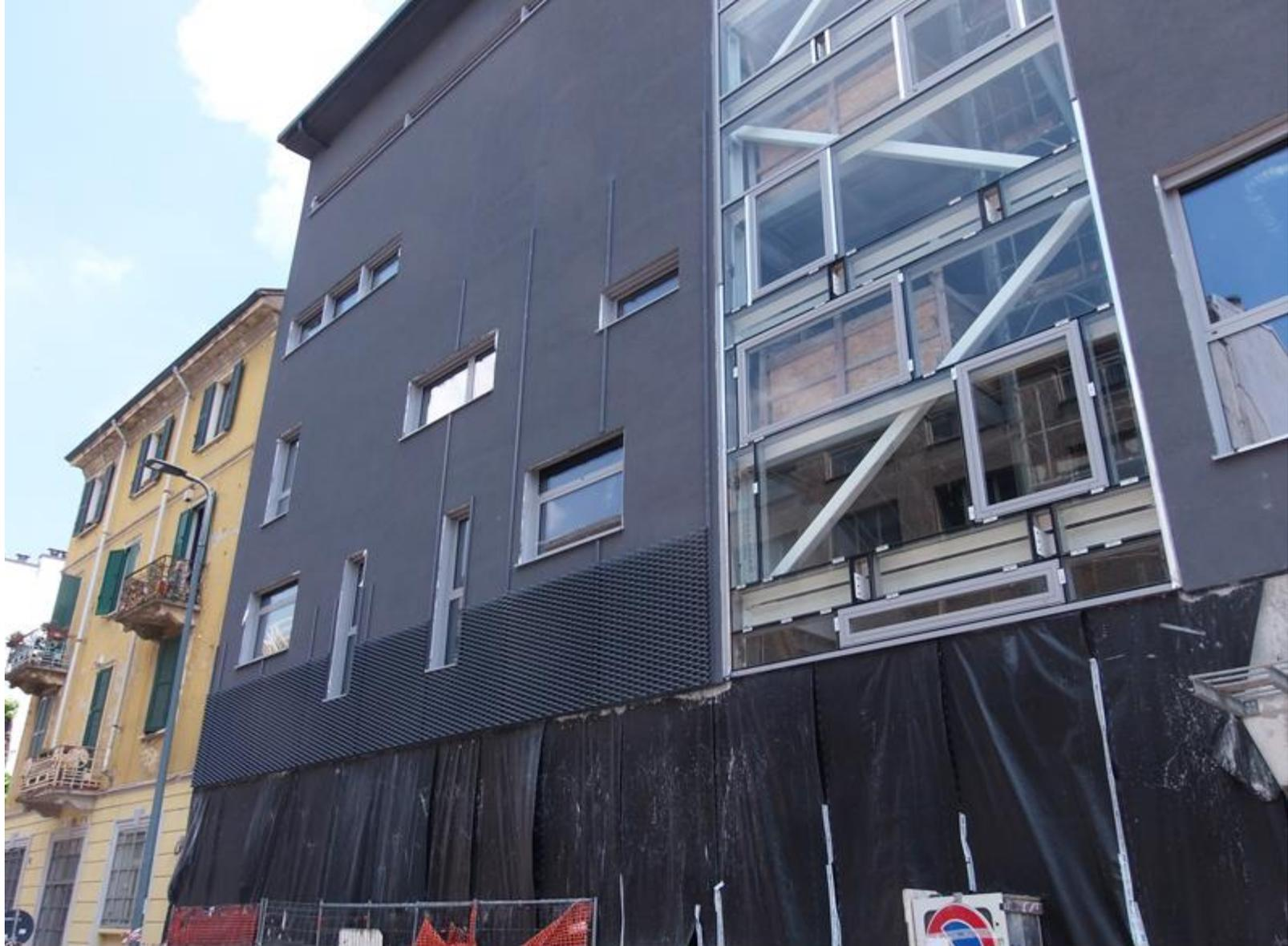
**POSA DI MONTANTI IN ALLUMINIO PER IL FISSAGGIO DEI PANNELLI IN LAMEIRA STIRATA DI METALLTECH**
