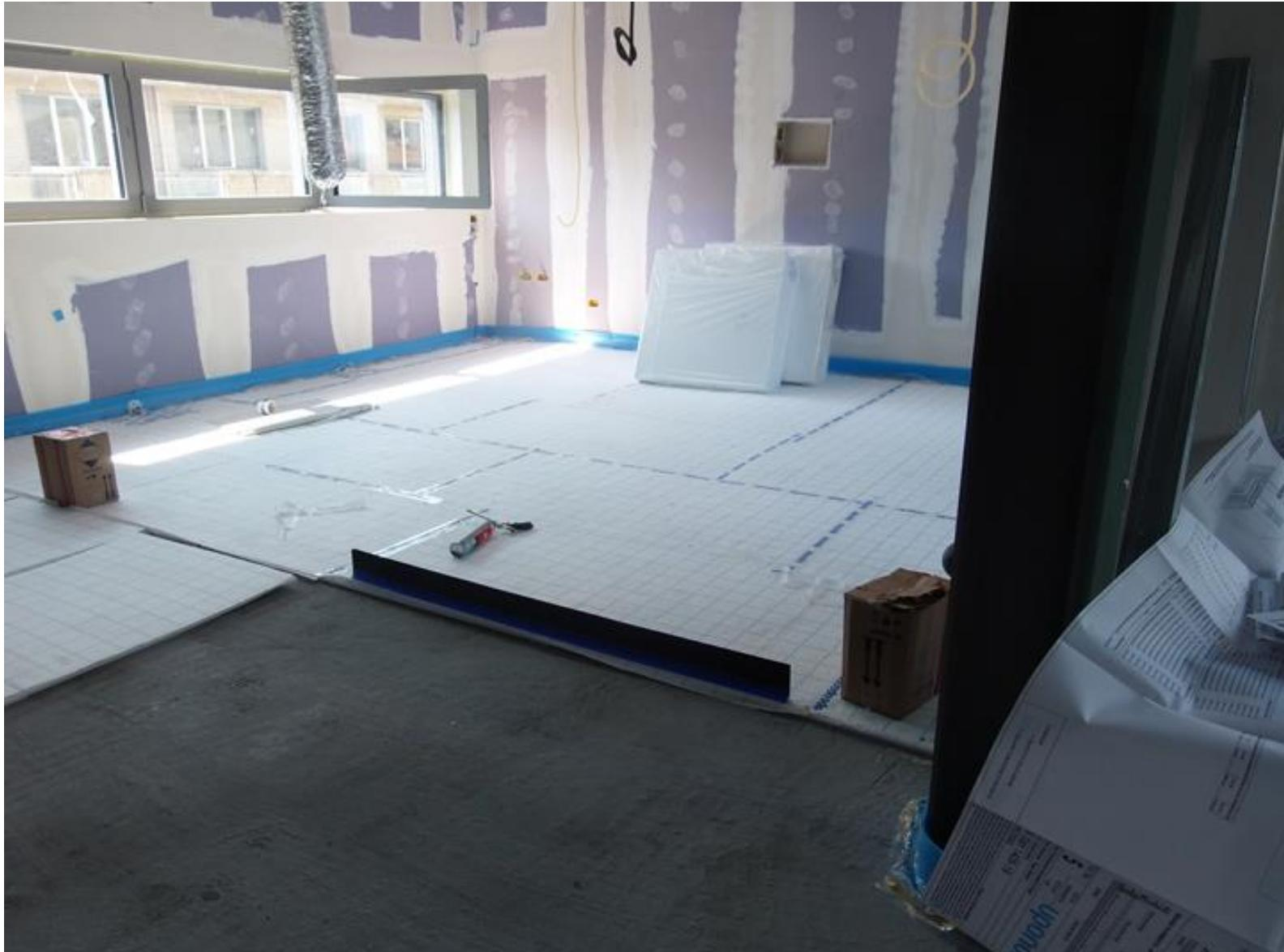
**POSA DI PANNELLI IN LANA DI ROCCIA E FINITURA CON DOPPIA LASTRA IN CARTONGESSO DI CUI LA PRIMA CON BARRIERA AL VAPORE E LA SECONDA KNAUF DIAMANT. POSA DI PANNELLI ISOLANTI RIBASSATI DA 1,5 CENTIMETRI PER LA POSA DEL PAVIMENTO RADIANTE UPONOR KLETT**
