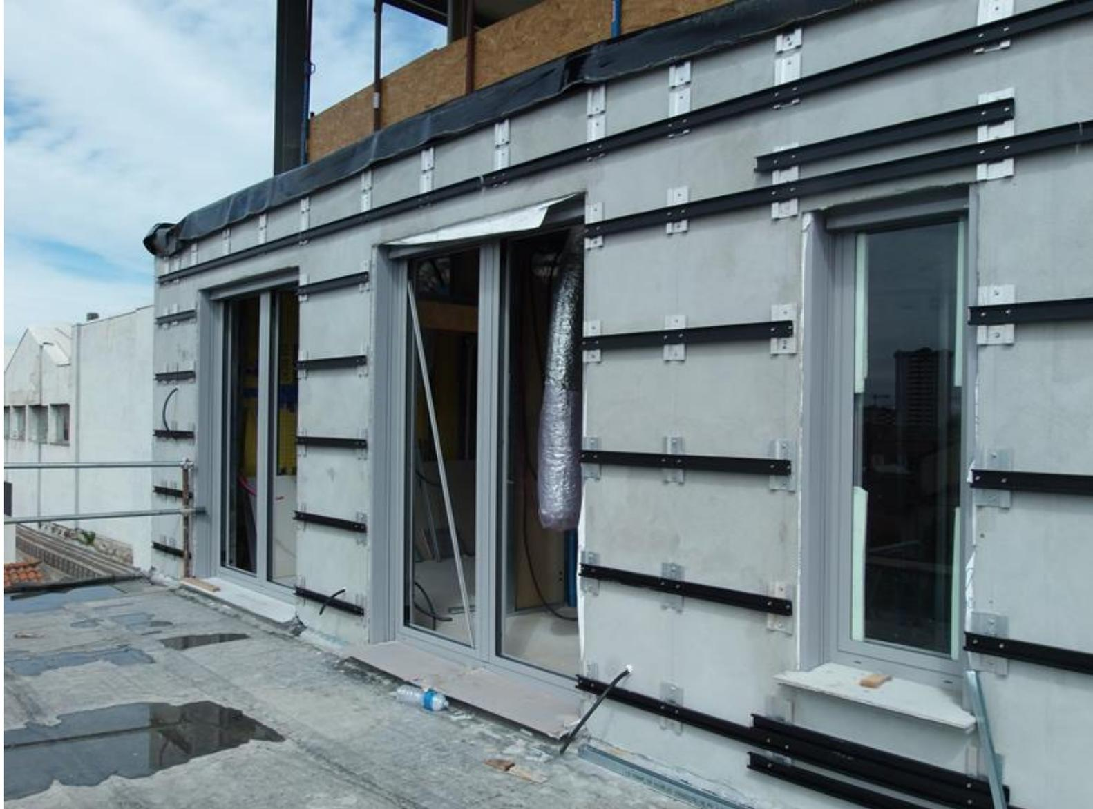
**MONTAGGIO DI STRUTTURA SECONDARIA DI SOSTEGNO DEI PANNELLI IN GRC. USCITA CORRUGATI ELETTRICI CON TAPPI IN GOMMA A TENUTA ALL'ARIA**
